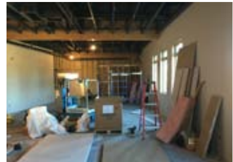
Drywall nearly complete in offices & youth room.
